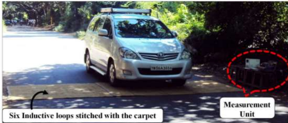
Figure 124: Inductive loop detector covering the entire road width.
