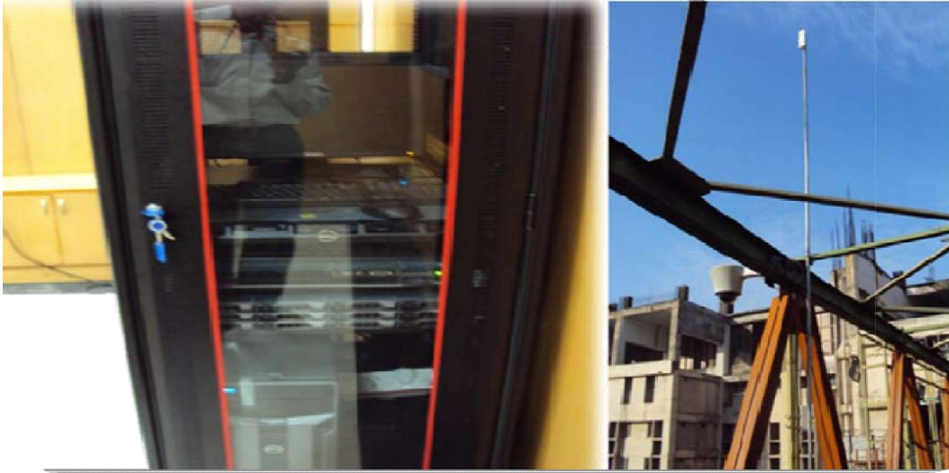
Figure 22: (a) Data storage server at IIT-M, (b) Wireless data communication antenna.
